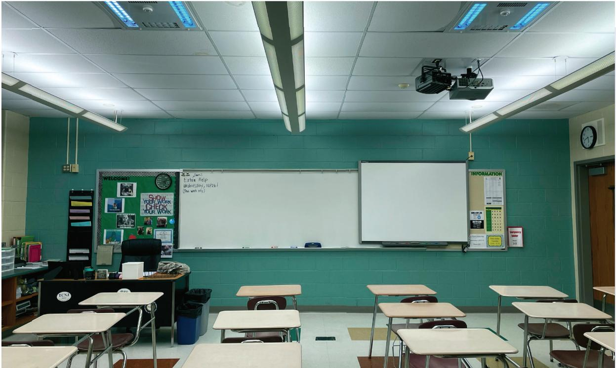
for the germicidal fixtures. A typical classroom, for instance, includes two hybrid UVC air-purifier and whole room disinfection fixtures with embedded McWong occupancy sensors. These are installed between the rows of regular direct/indirect pendant lighting and operate on the same electrical circuits.
